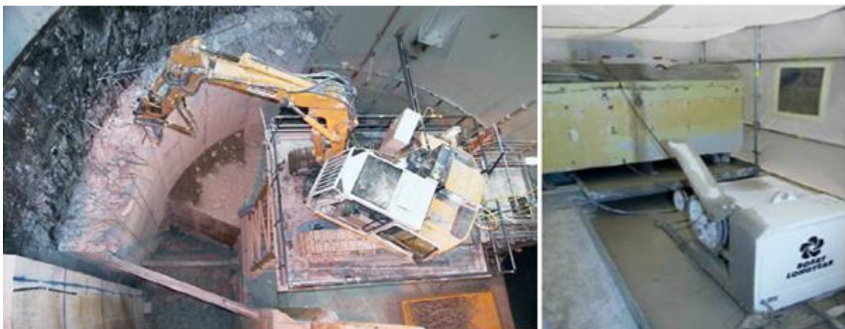
Figure 4-25: Removal of large quantities: left excavator, right: wire rope
