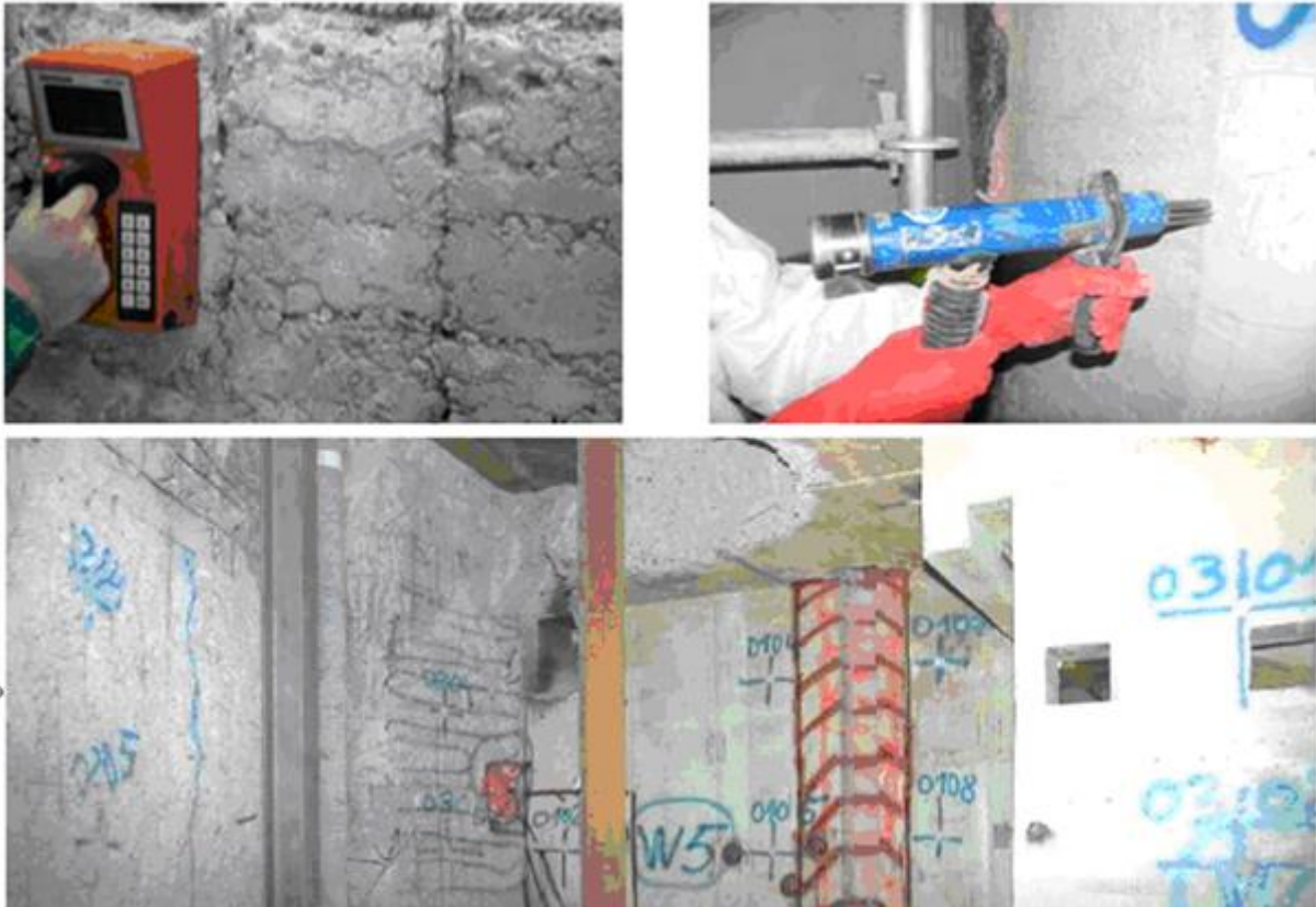
Figure 4-21: Concrete in controlled area during radiological characterization
