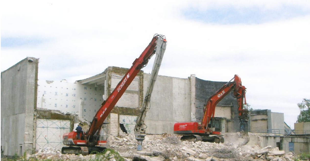
Figure 4-28: Conventional dismantling of the building structures
