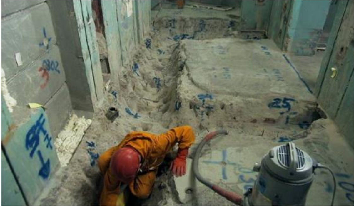
Figure 4-24: Removal of deeper contamination
