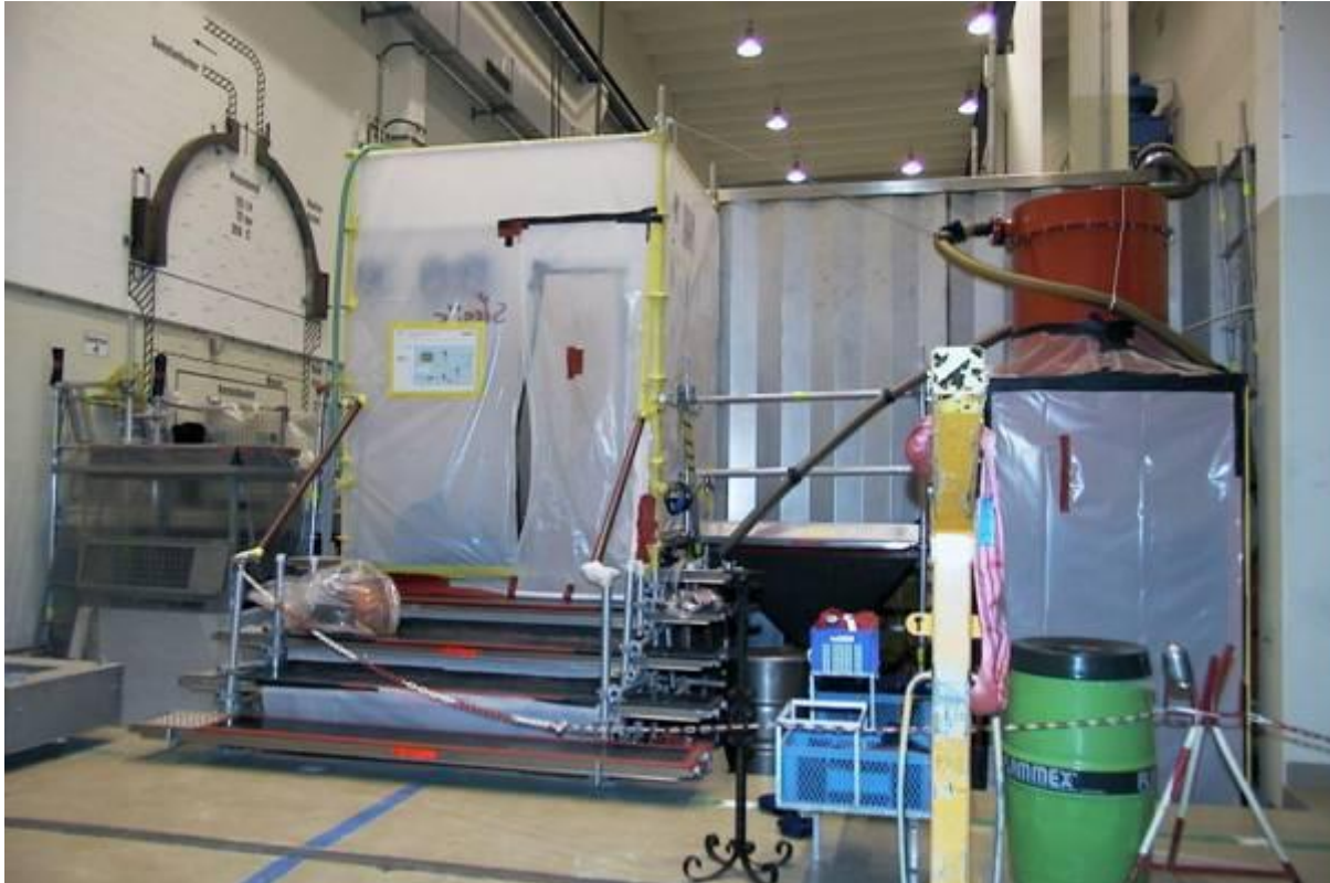
Figure 4-10: Blasting caisson at Kahl NPP
