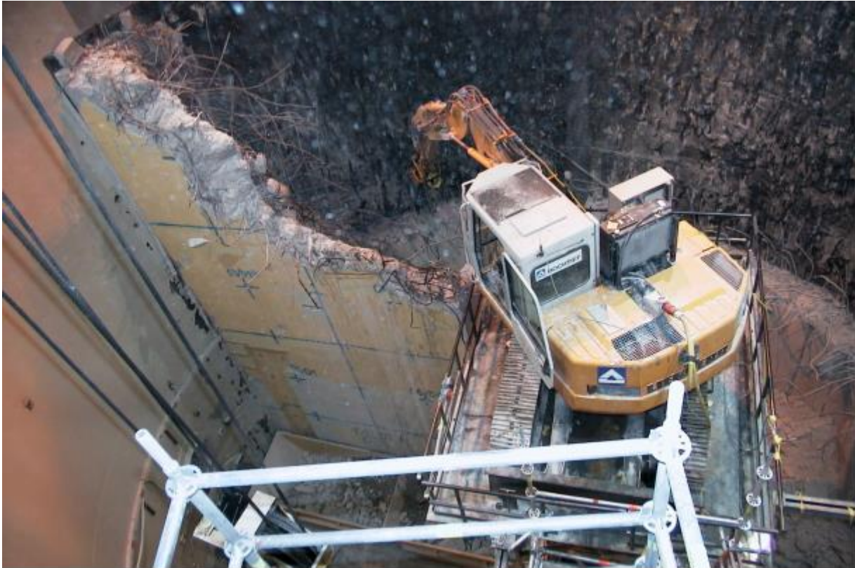
Figure 4-16: Dismantling of concrete inside containment
