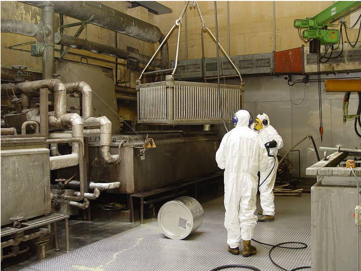
Figure 4-11: Chemical decontamination [reference EWN]
