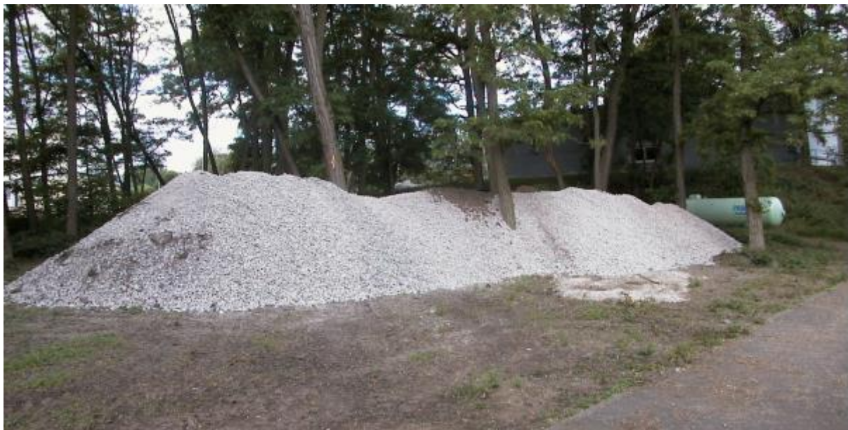
Figure 4-18: Free released concrete to be used for filling of pits
