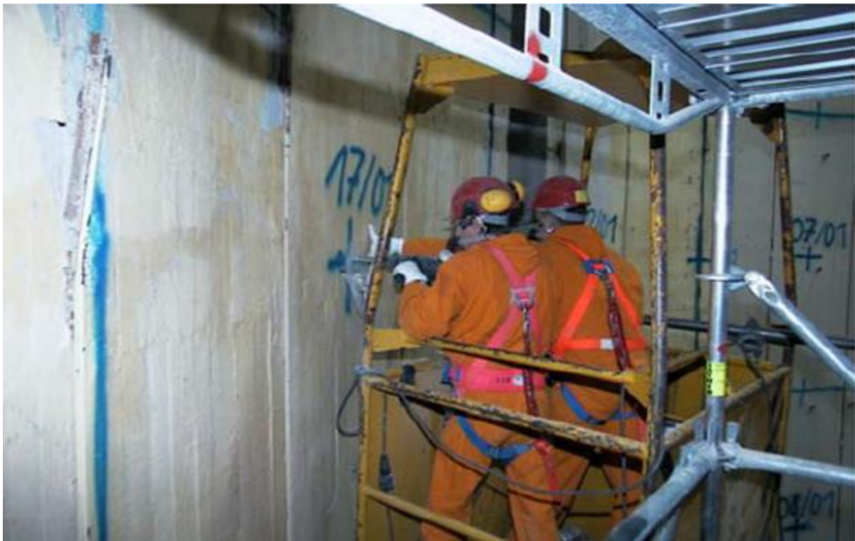
Figure 4-23: Preparation of scarification: removal of dowels
