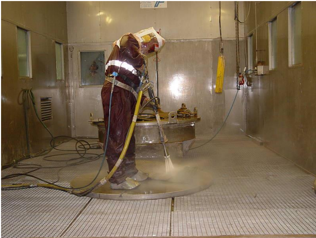
Figure 4-8: Wet decontamination by high pressure water [reference EWN]
